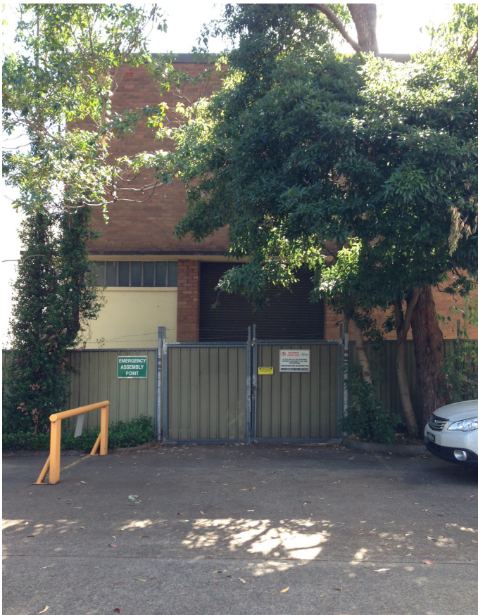
Figure 26 - View of Entry to Sydney Water building
