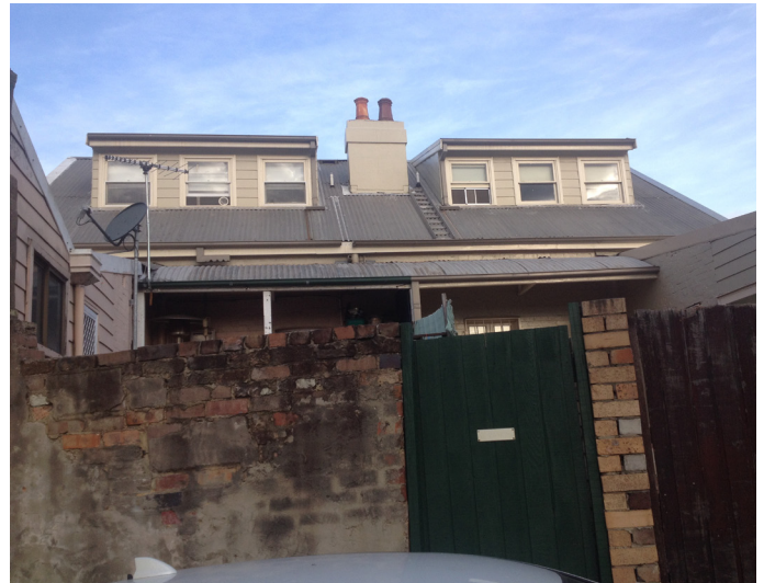
Figure 28 - Rear of heritage items from McPherson Lane
